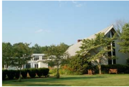
Courtesy of St. Paul's Church in Bedford St. Paul's Church being built in Bedford in 1958 (top), and St. Paul's Church today
