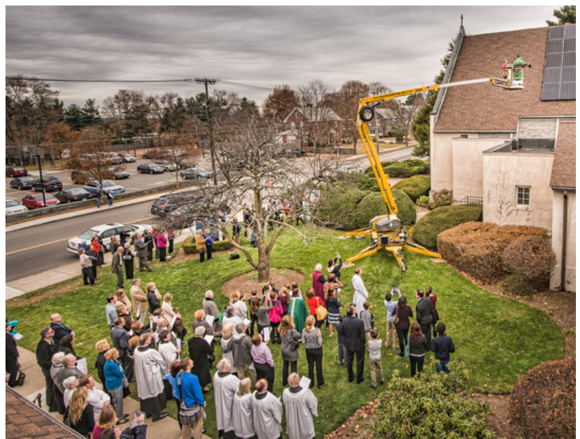
A blessing of a church roof's solar panels.
